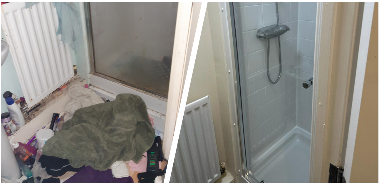
Void property – before and after
